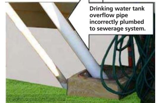
Figure 3: Examples of a stormwater pipe illegally connected to the sewerage system.
